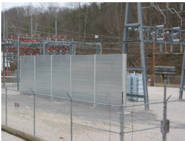
Engineered sound control wall installed
