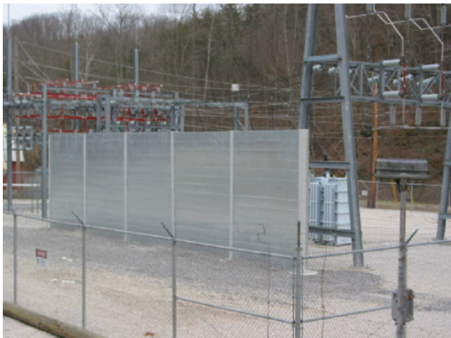
Engineered sound control wall installed
