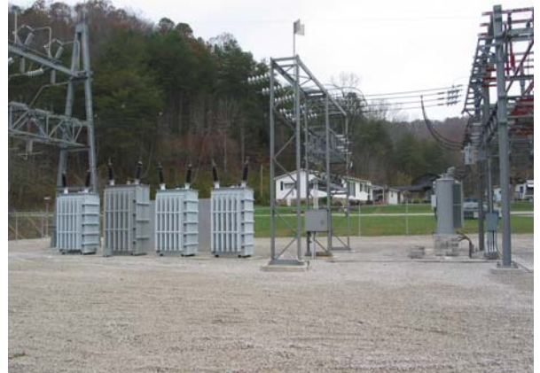
Transformer station near residential house before
