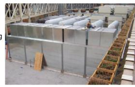
Third, because the "generator housing" or sound enclosure is technically a temporary or moveable structure, permitting is simpler versus constructing a fixed building to house the genset units.
