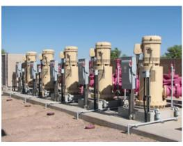
Below are several examples of Well Pump Sound Enclosures with silenced ventilation, removable panels and complete enclosure lift-off option.
