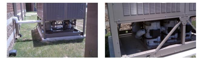
eNoise Control wrapped, with acoustical blankets, a quantity of ten (10) scroll compressors on the two chiller units. In addition to the compressors, the chiller units piping and oil separators were also wrapped with the acoustical blankets.
