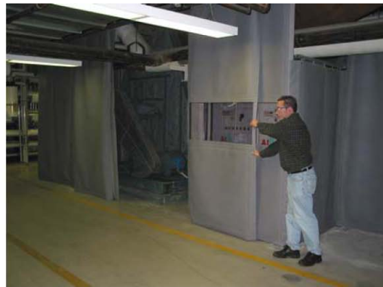
Fan shown with sliding access sound curtain
