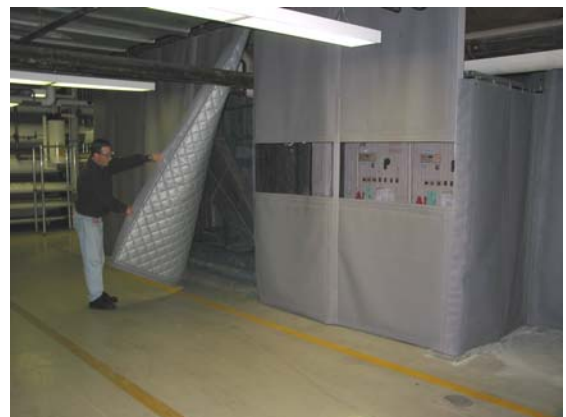
Modular sound curtains used on double sliding track.
