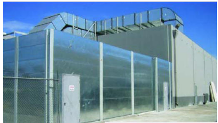
Sound wall used to control outdoor noise
