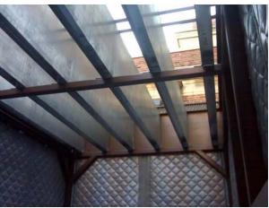
The solution was to provide adequate access to service the condensing units, to not restrict airflow allowing the units to run properly, and to stop the fan noise from reflecting off the nearby structures. Sound curtains were used to enclose the top of each unit attached to a tubular steel frame. Vertical baffles or louvers were set above the condenser fans and sound curtain structure to create a large silencer. The result was total success on all criteria.
