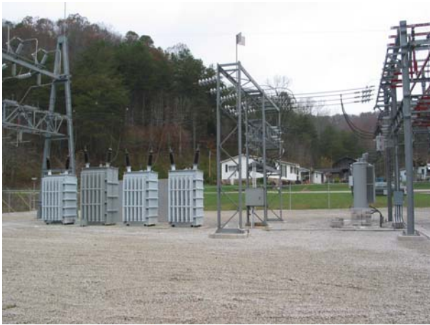
Transformer station near residential house before
