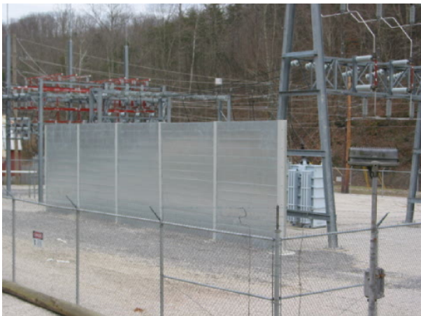
Engineered sound control wall installed
