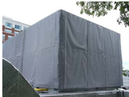
Perimeter Blanket on Fence
